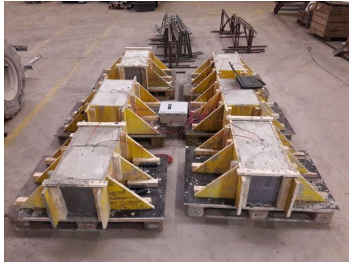
Figure 6: Koralmtunnel KAT3 - Production of specimen for in situ shrinkage and creep tests.
