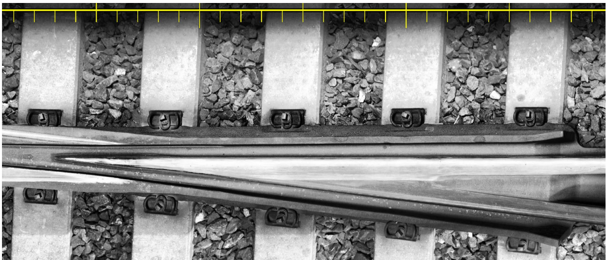
Figure 13 - Frog of one of the project turnouts
